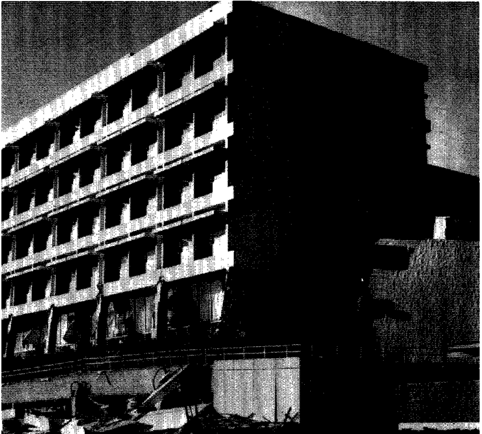
Figure 19.2.5 Olive View Hospital building. The shear walls in the upper four stories did not extend to the lower two stories. (From K. V. Steinbrugge Collection, courtesy of the Earthquake Engineering Research Center, University of California at Berkeley.)
