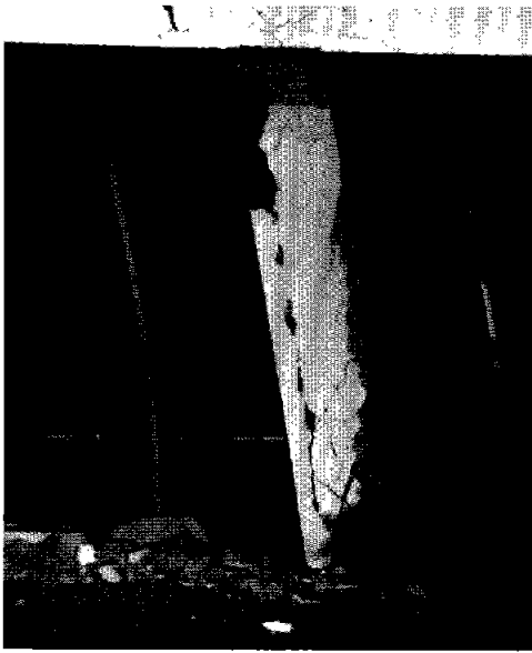
Figure 19.2.8 Large permanent deformation of a spirally reinforced column of the Olive View Hospital building. (From K. V. Steinbrugge Collection, courtesy of the Earthquake Engineering Research Center, University of California at Berkeley.)
